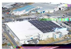
Figure 9: Nagoya Works 1: 750-kW power generation facility
