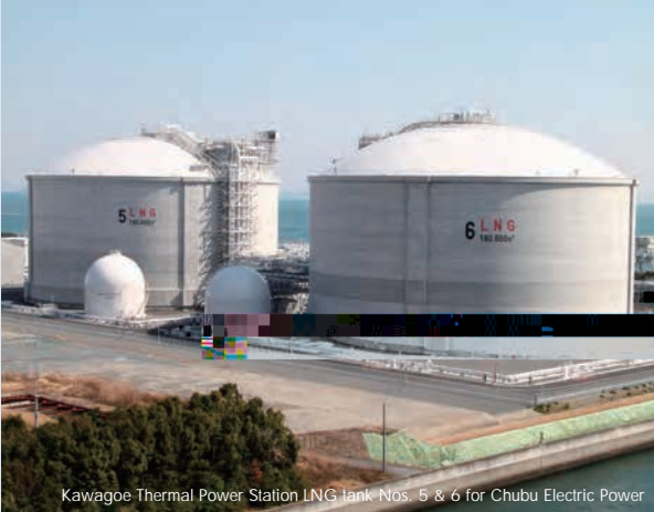
Kawagoe Thermal Power Station LNG tank Nos. 5 & 6 for Chubu Electric Power
